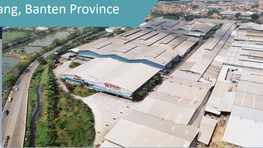
Kapuk Plant (Heat Exchange)
